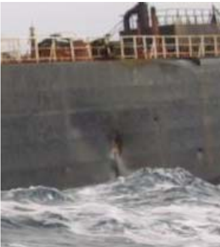
Setting in of shell plating at Frame 85 on port side of the vessel
