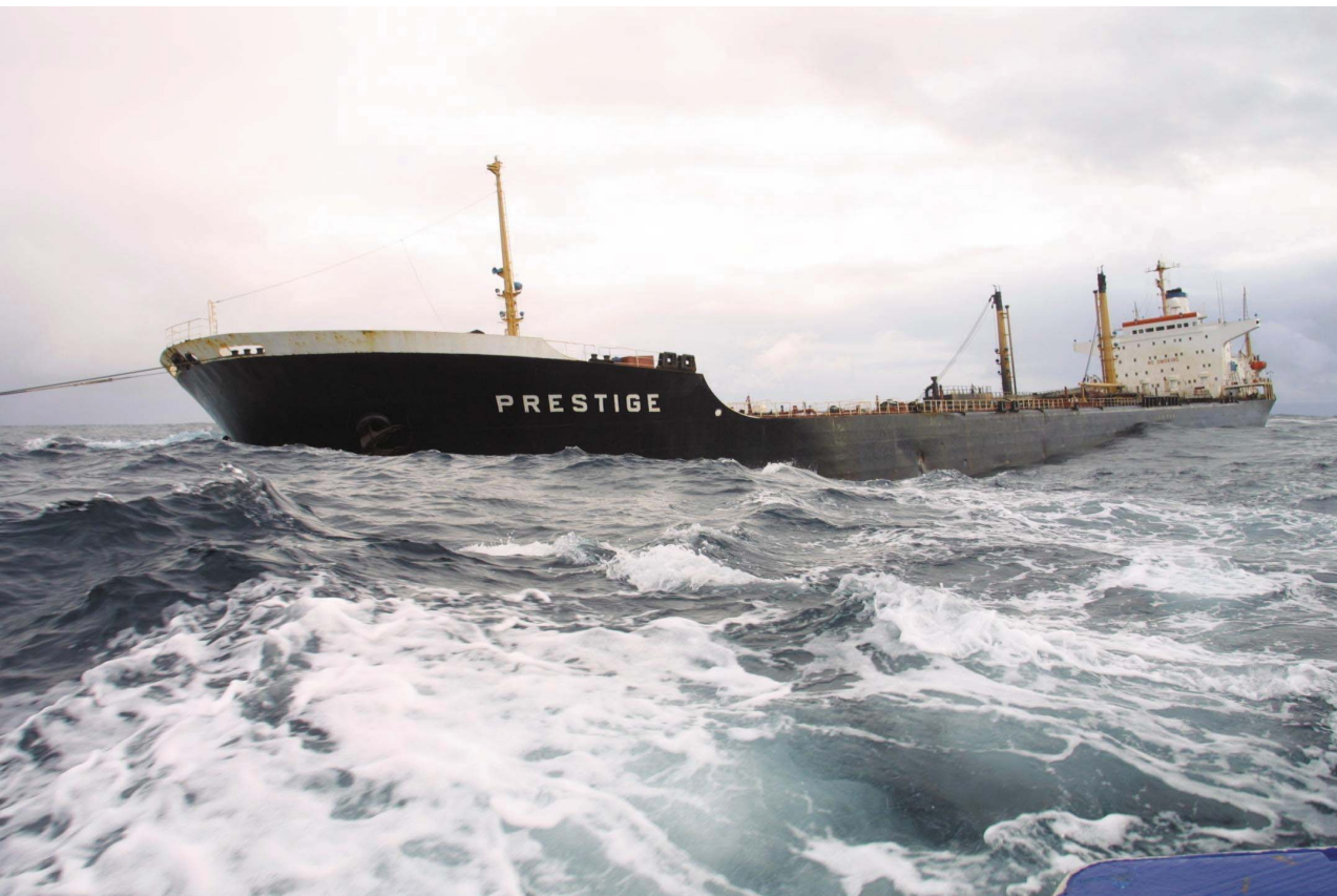
General views of the port side showing setting in of shell plating (See enlarged views in Figure 11)
