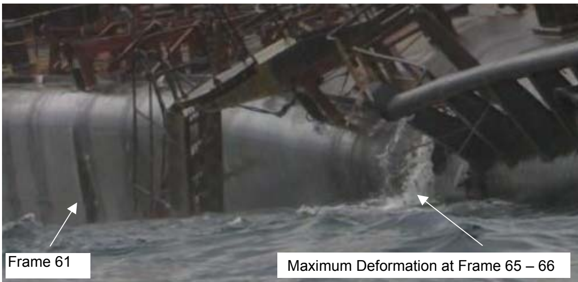
Main deck edge from aft end of 3 Starboard wing tank (Frame 61) to mid length of tank (Frame 65)
