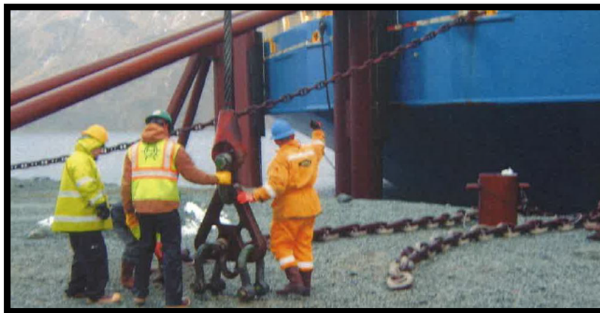
Figure 14: Preparing to Connect the Towing Plate to the Bridle Legs (Photo courtesy of GL Noble Denton, Mr. █████)
