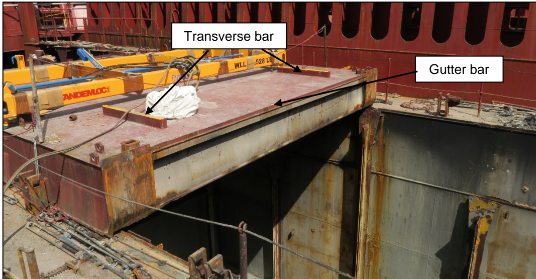
Figure 19: Cargo hold 1, bay 1, gutter bar and transverse bar
