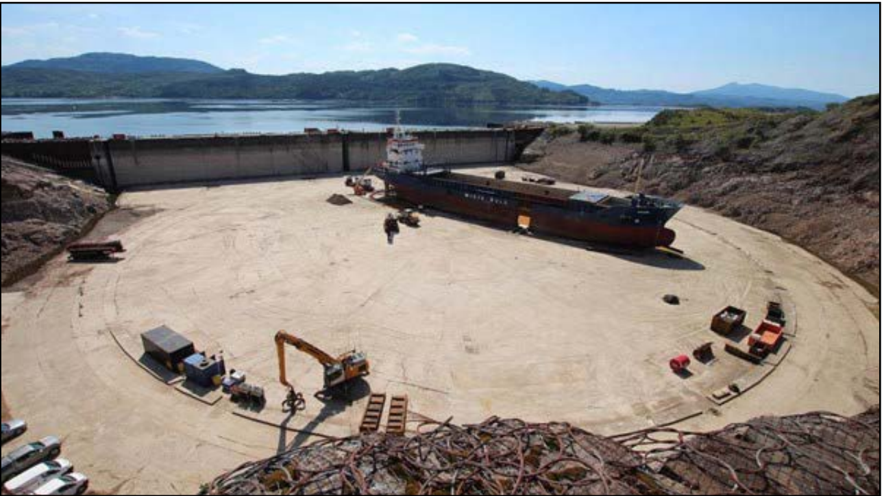
Figure 7: Kaami in the Kishorn facility
