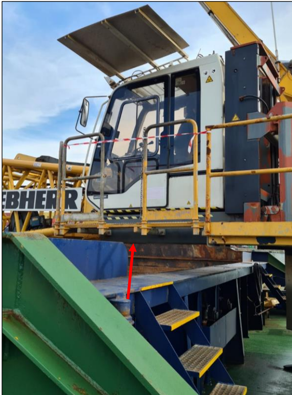
Figure 6: Access to the crane from starboard side
