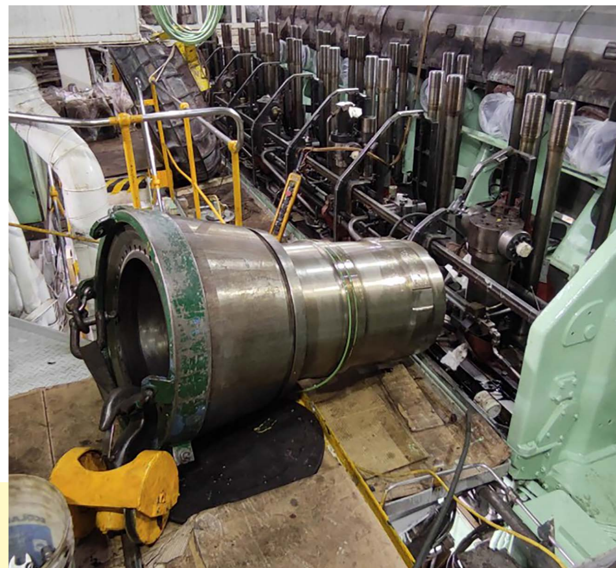
Figure 2: Position of cylinder liner after wire failure
