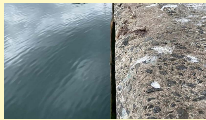
Figure 2: The sloping quayside
