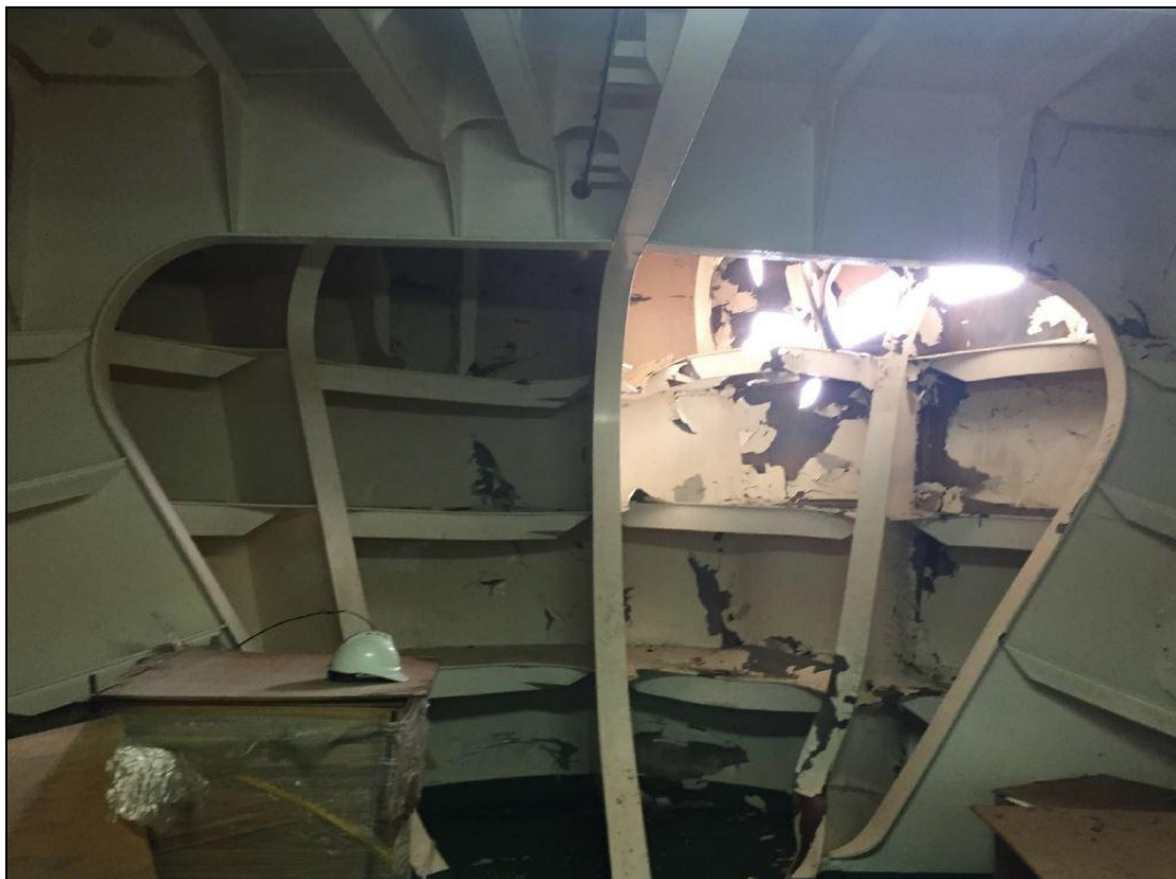
Figure 18: Internal view of damaged shell plating on the starboard bow
