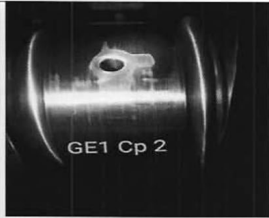
Crank pin with wear ridge condition
