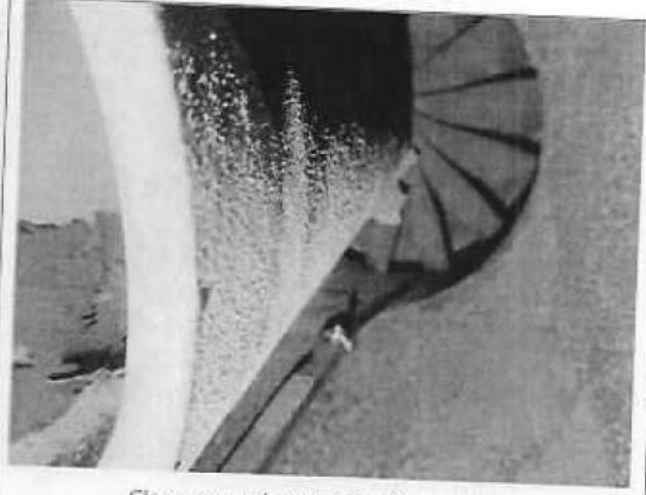
Clearance taken during dismantling
